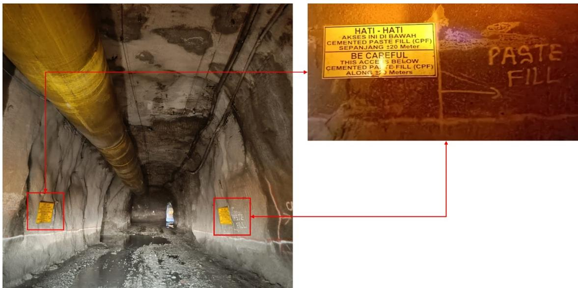
**Figure 6** Cemented paste fill drift condition looking south after development and with signage
