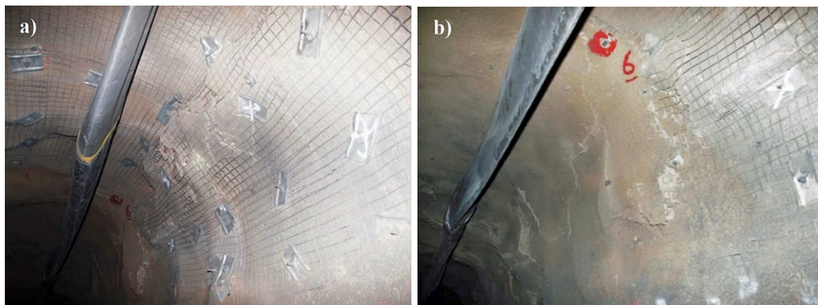
Figure 26 (a) Fibre-reinforced shotcrete; (b) Mesh-reinforced shotcrete (Drover & Villaescusa 2015)
