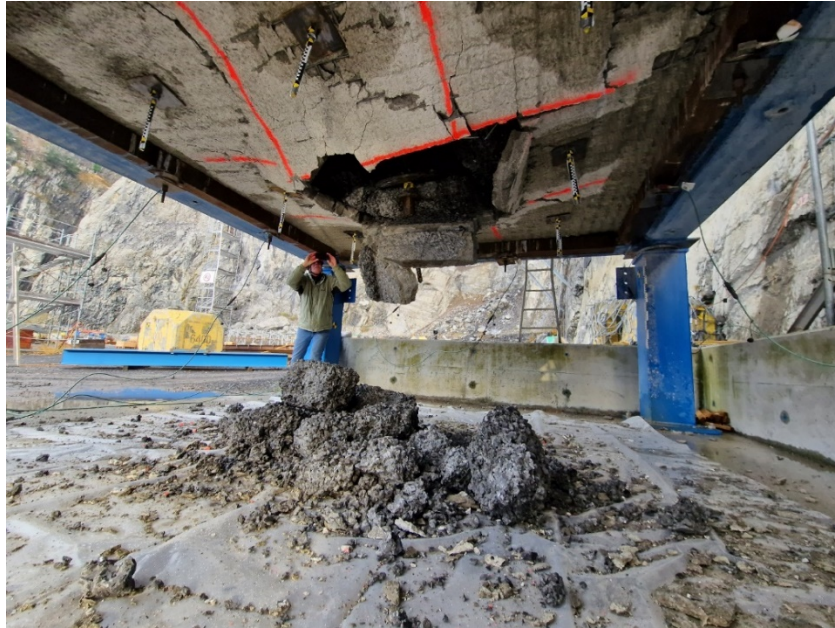
Figure 10 Failed centre bolt and ruptured mesh after testing
