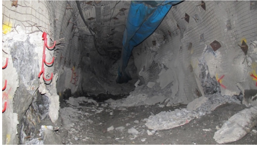
Figure 5 Seismic event occurred on 3 October 2018, at F7775NOD showing floor heave
