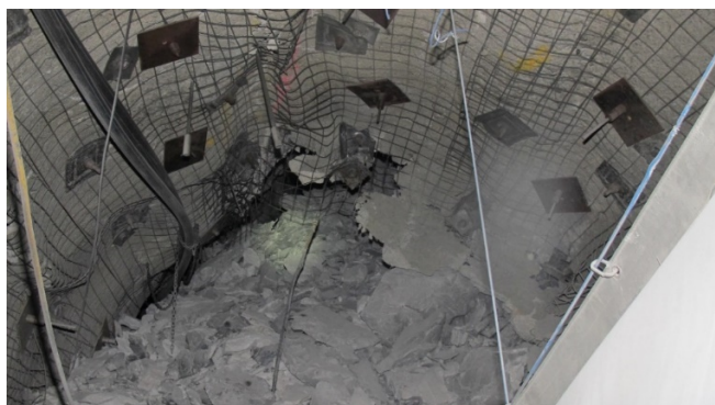
Figure 4 Fall of material from the backs, south of the paste barricade. Note how fractured the material is
