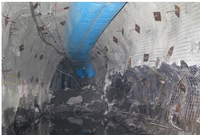
Figure 2 Rehabilitated area following a seismic event occurred on 13 August 2018, at F7775NOD
