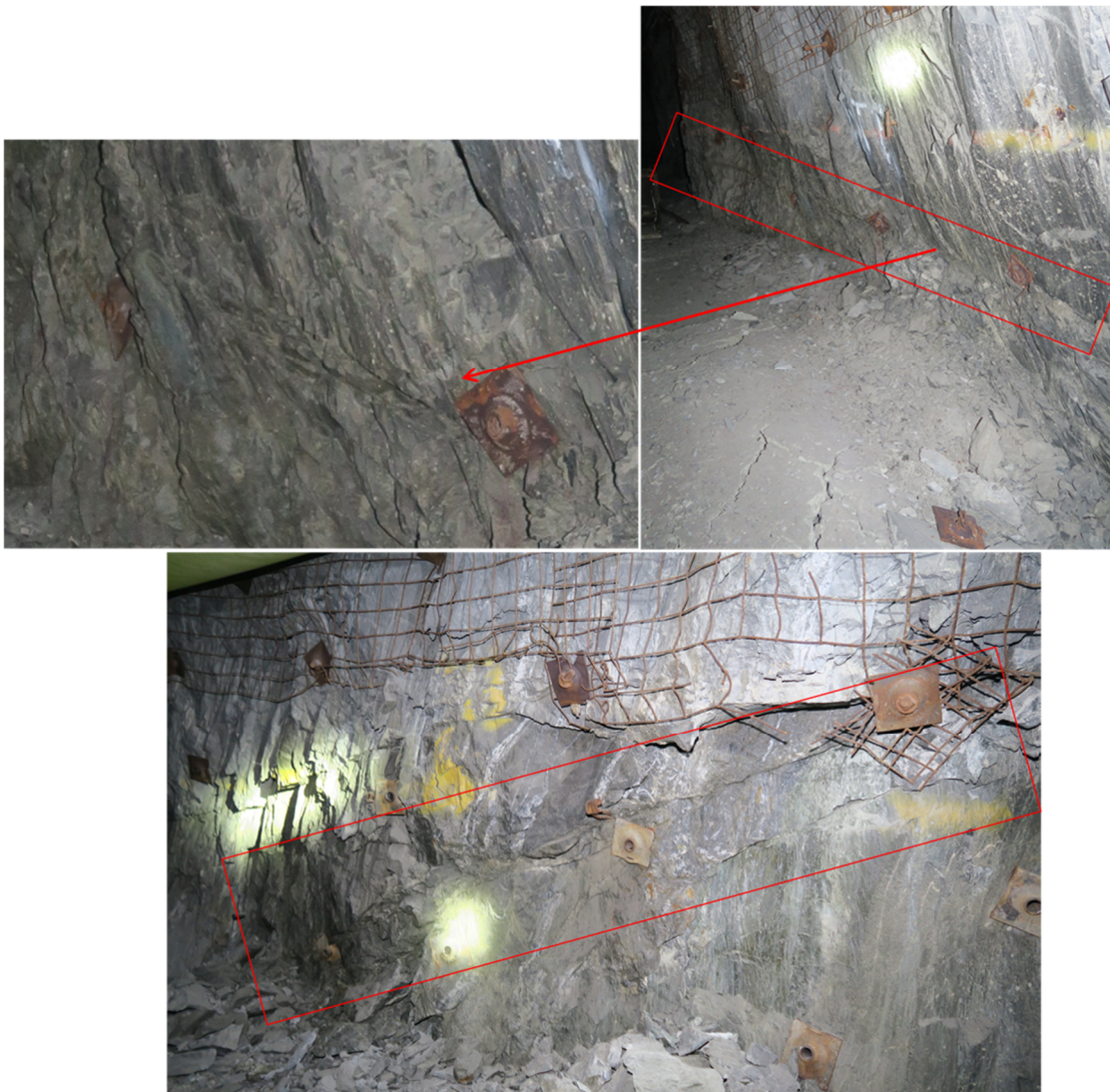
Figure 2 Photo of low-angle structures on walls of 1,185 mbgs sill at the floorburst location
