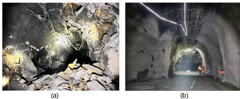
Figure 20 Repairs to sector 2: (a) Post-rockburst condition; (b) Repair work completed
