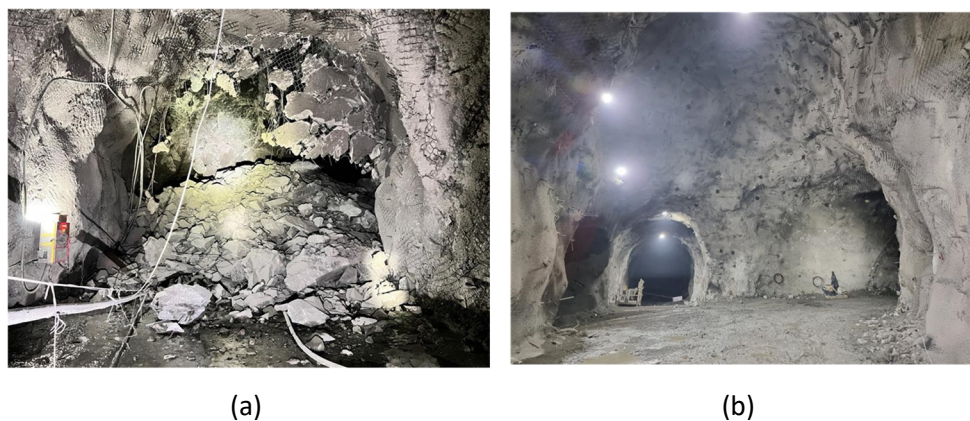
Figure 18 Rehabilitation in sector 1: (a) Post-rockburst condition; (b) Rehabilitation completed
