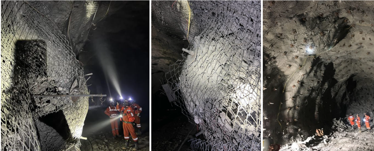
Figure 16 Photographic register from the ground inspection after a seismic event. Deformation is evident in the contour of the excavation
