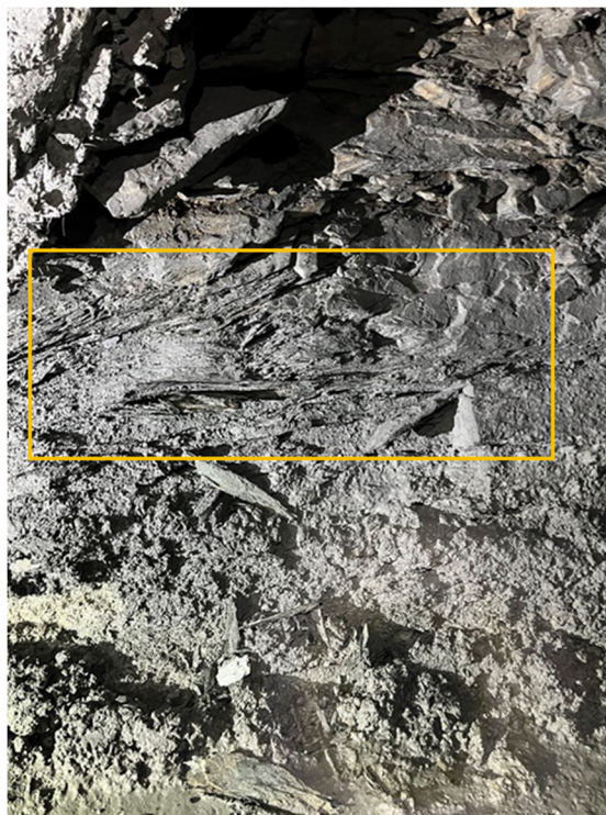
Figure 6 Photograph of the banded iron formation contact in a drive sidewall, showing the laminated graphitic zone, evidently weak in shear
