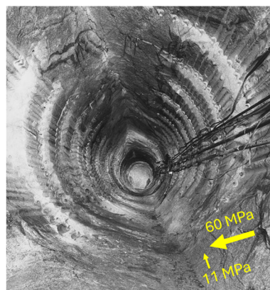
Figure 2 V-shaped notch failure around the mine-by experiment tunnel at 420 Level of the URL (after Read et al. 1998)
