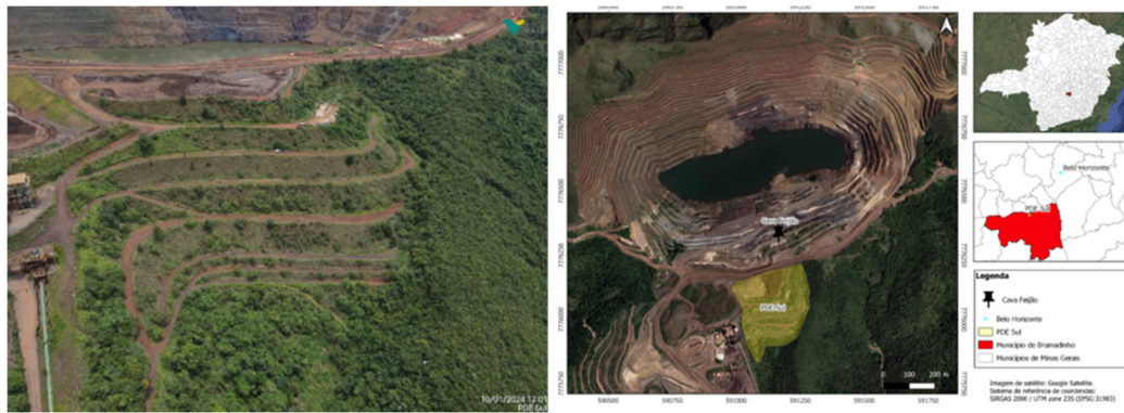
Figure 1 View of PDE Sul and its location within the Córrego do Feijão mine
