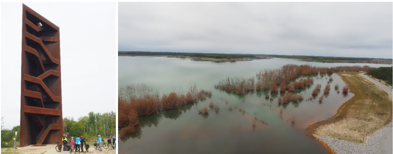
Figure 1 The Rusty Nail installation and viewpoint at the nexus of several cycle routes where three pit lakes meet, with views from the top (source: Peter Whitbread-Abrutat)
