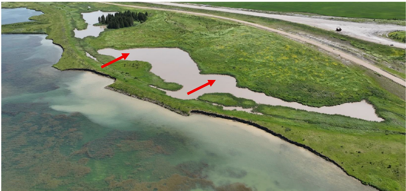
Figure 11 East portion of Southeast Dyke. Red arrows indicate areas of erosion and ponded water downstream of the dyke (downstream direction is towards top of photo)
