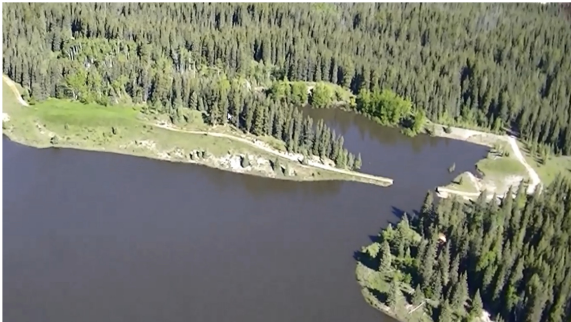
Figure 2 Klein Lake Dam failure in 2013 showing breach of Cofferdam and Main Dam impounding released water
