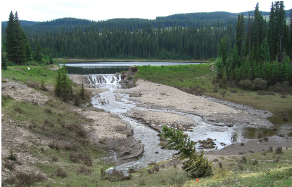
Figure 3 Cofferdam breach viewed from Main Dam in July 2013
