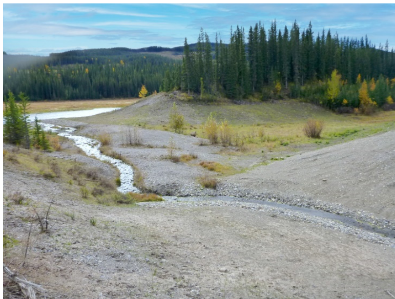
Figure 6 Cofferdam removed in September 2020, abutments of removed Main Dam in foreground
