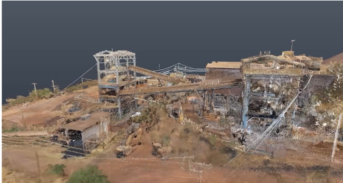
Figure 7 Laser scan representation of an industrial structure at the Córrego do Feijão Mine, developed as part of a digital twin model
