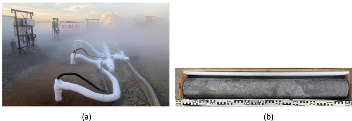
Figure 5 (a) Seese-East freeze plant (2023); (b) Freeze drill core from a depth of 27–28 m (Reinhardt et al. 2024)
