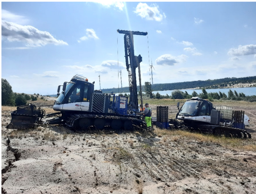
Figure 2 Use of light, mobile drilling technology for the Seese-Ost inner dump (LMBV mbH & BIUG GmbH 2022)
