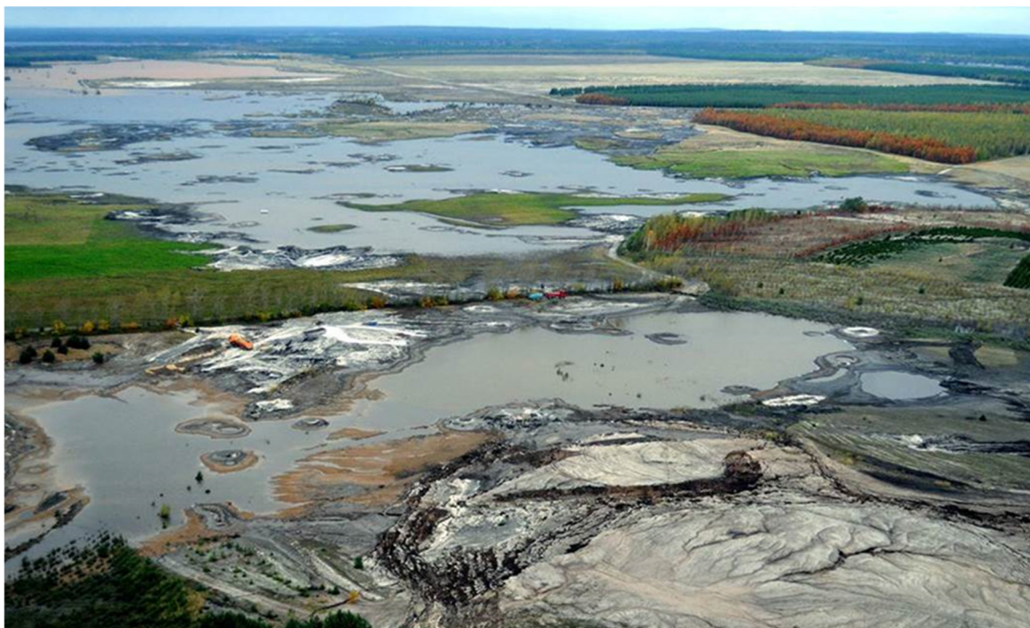
Figure 1 Soil liquefaction at the Spreetal inner dump on 12 October 2010, with an impacted area of approximately 160 ha (Scholz & Mühlig 2019)
