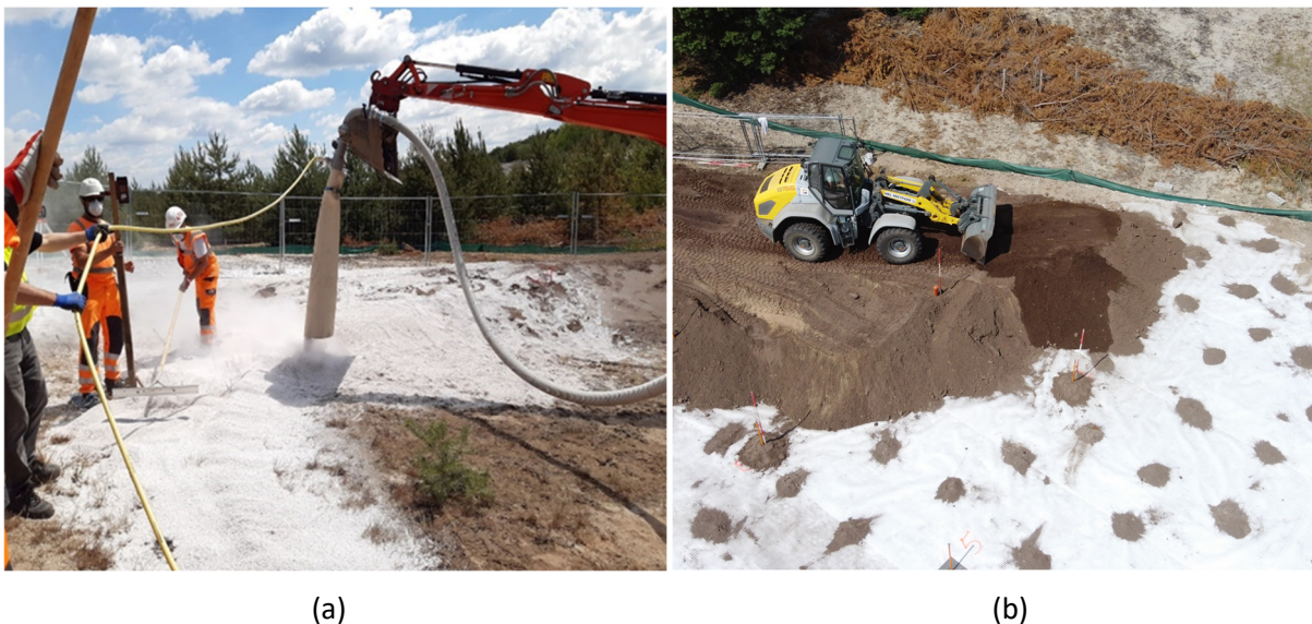
Figure 8 (a) Placement of perlite in the test field; (b) Covering of the perlite area with soil material (Soltau et al. 2025)
