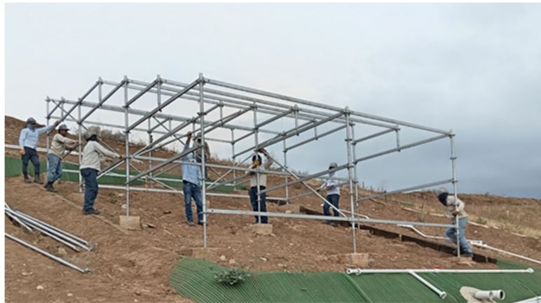
Figure 8 Installation of the scaffolding that forms the structure of the simulation system
