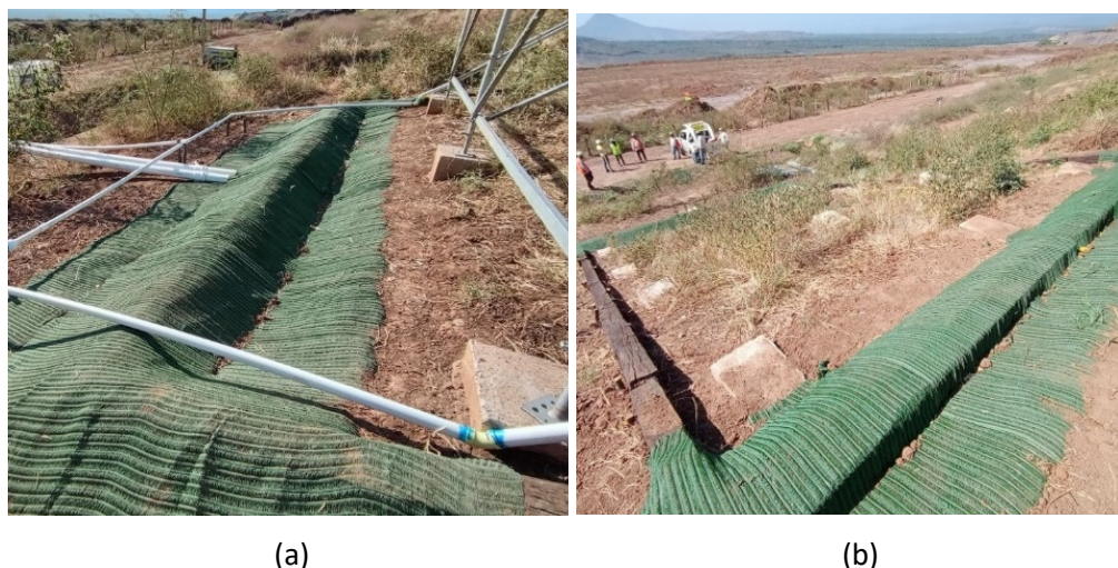
Figure 7 Details of the erosion cell. (a) Bottom ditch of the erosion cell; (b) Wooden barriers
