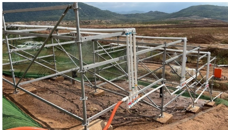
Figure 9 Typical view of an erosion cell
