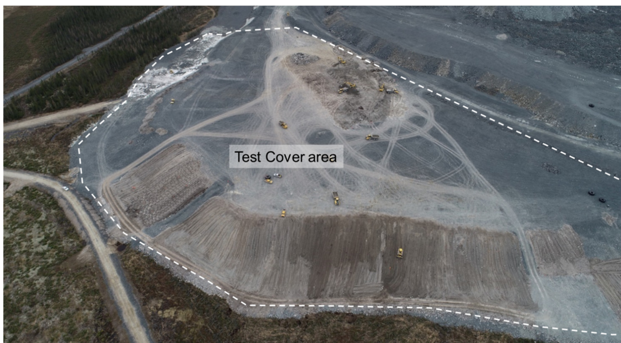
Figure 1 Test cover in May 2019 showing construction and cover material placement. Dashed outline represents the test cover project area
