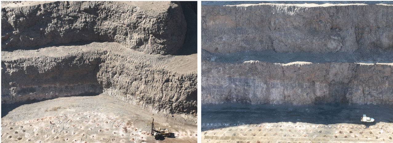
Figure 15 Examples of slope performance with recommended bench–berm parameters at Big Mack
