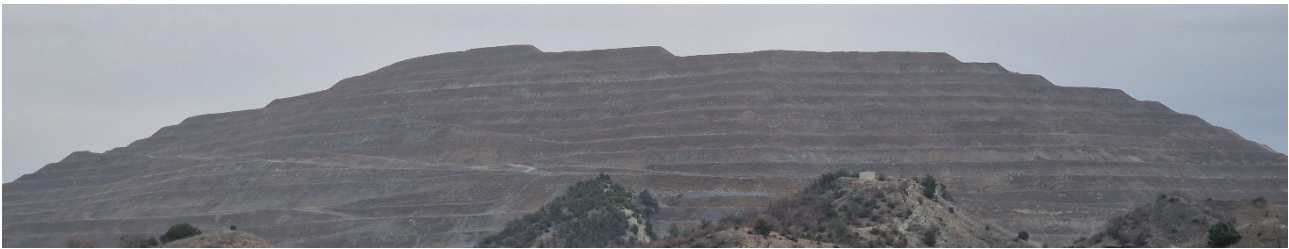
Figure 4 Photo of the western slope of the waste dump
