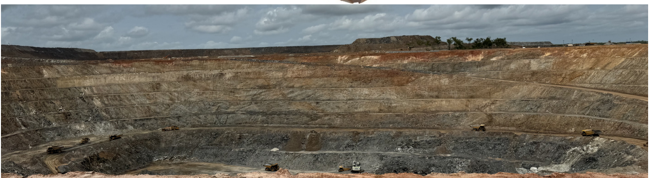
Figure 7 Aerial view of the site and an overall photo of the upper west wall in December 2023
