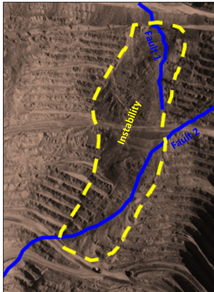
Figure 8 Major-scale instability at the pit wall
