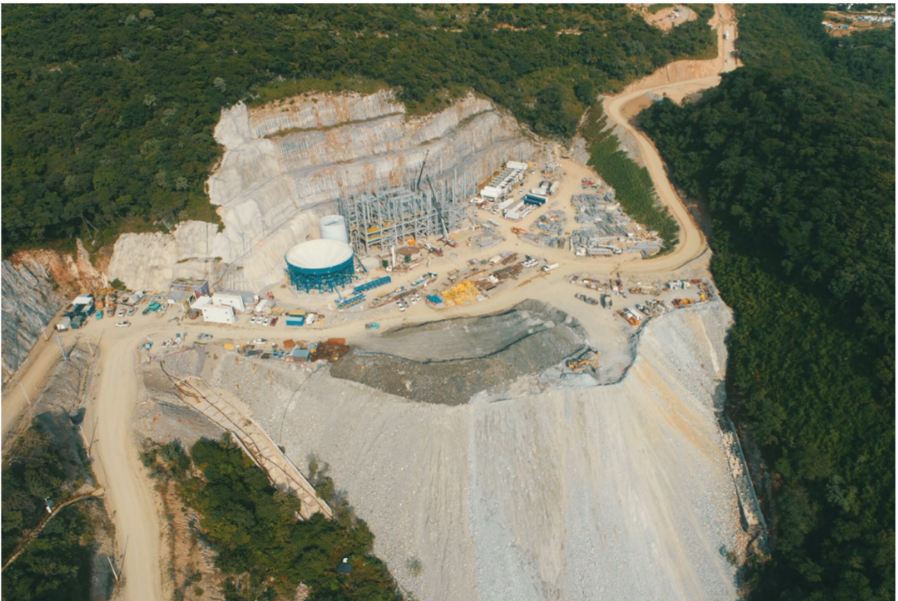
Figure 6 Media Luna paste plant construction (15 October 2024, courtesy of M3 Engineering)
