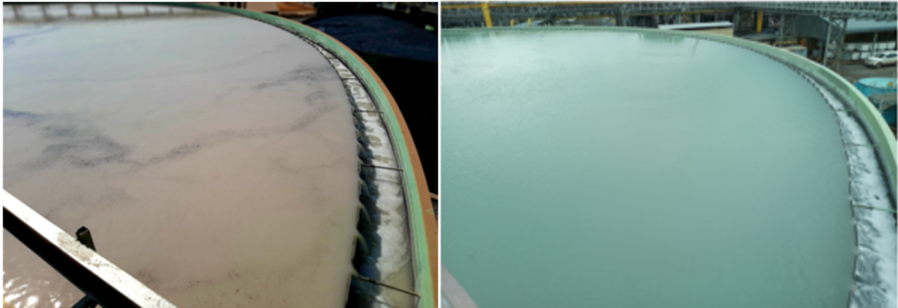
Figure 6 Tailings thickener overflow before and after changes
