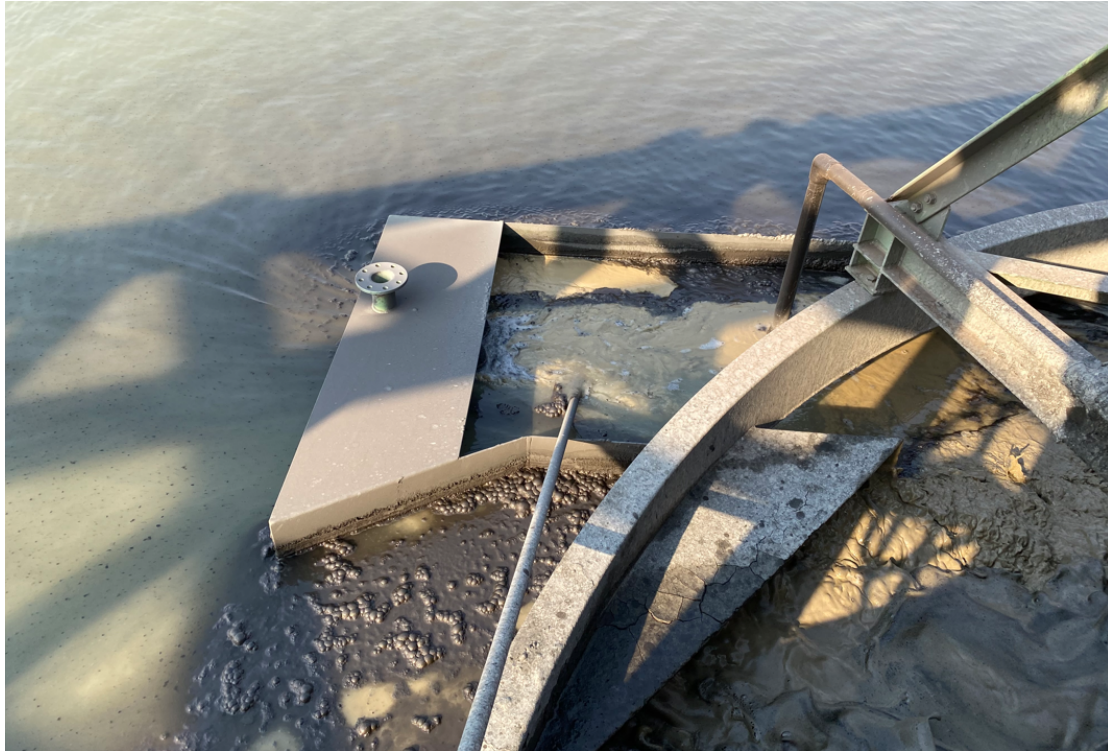
Figure 10 Feedwell dilution channel in operation
