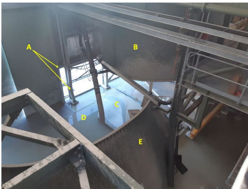
Figure 4 Example slurry tank failure (WorkSafe 2019)
