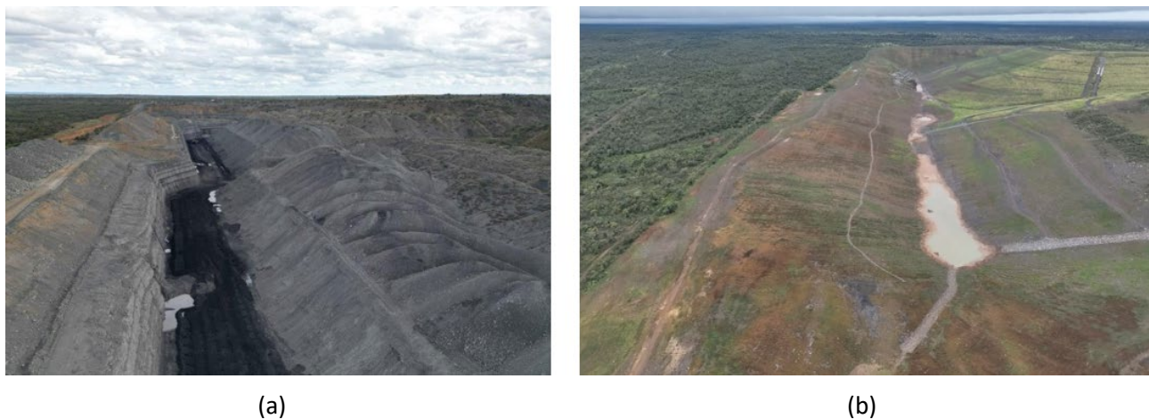
Figure 4 Ramp 10 (Eastern Creek). (a) October 2022; (b) February 2026
