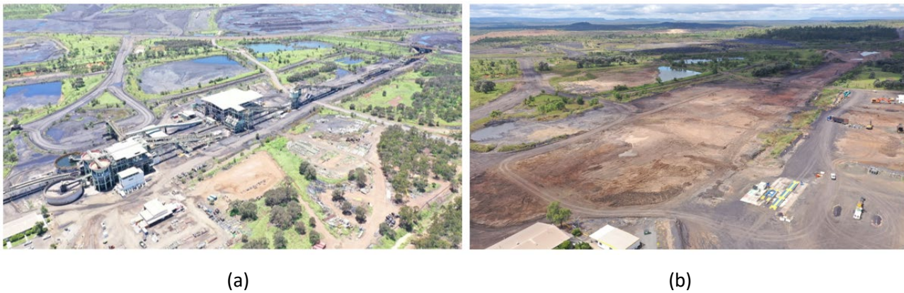
Figure 6 CHPP decommissioning (Main Deposit). (a) 2020; (b) 2025
