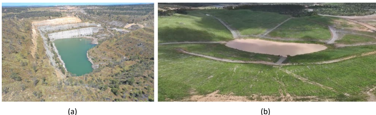
Figure 5 Ramp 2 Southern Underground (Main deposit). (a) August 2022; (b) February 2026
