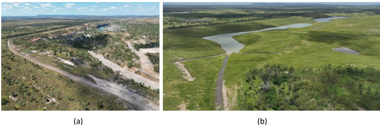
Figure 3 Ramps 15–17 (Suttor Creek). (a) April 2023; (b) February 2026
