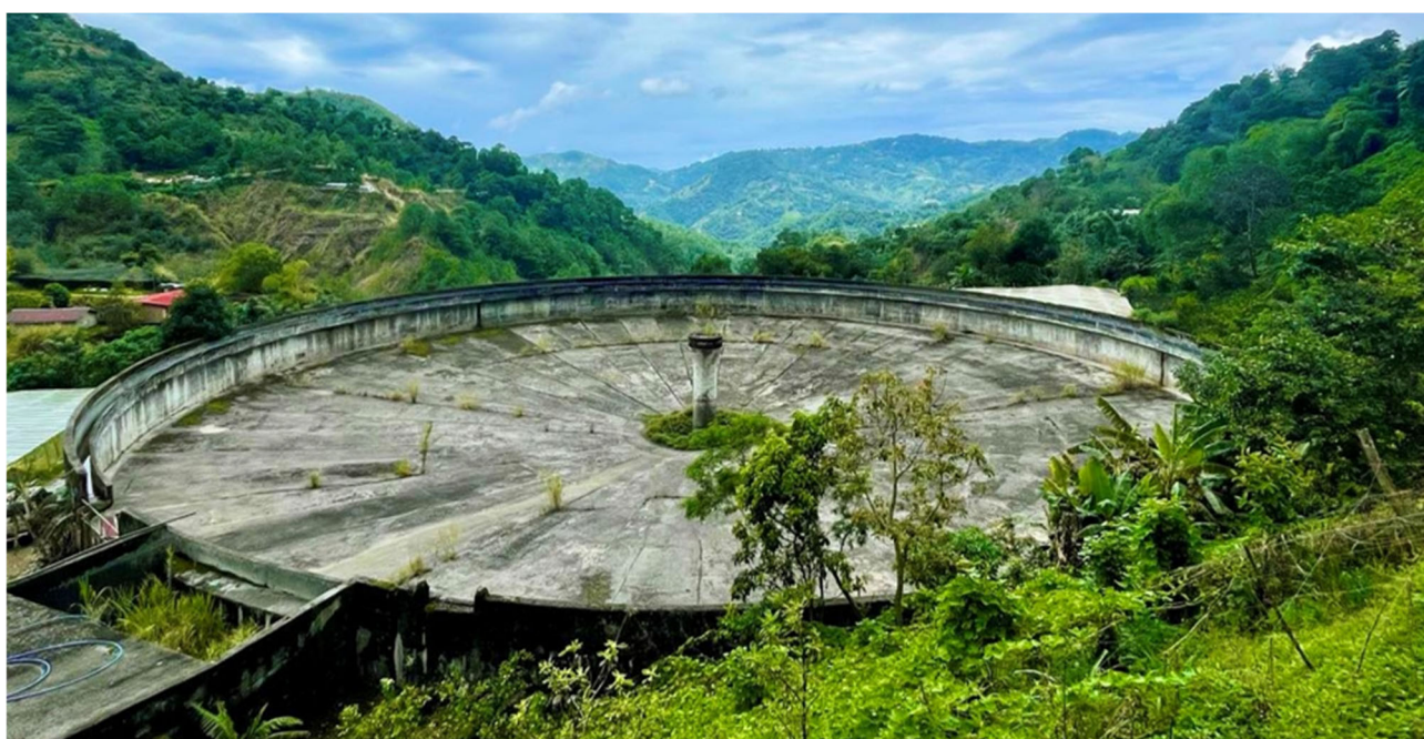
Figure 1 Abandoned 200 ft-diameter tailings thickener left at the mine site
