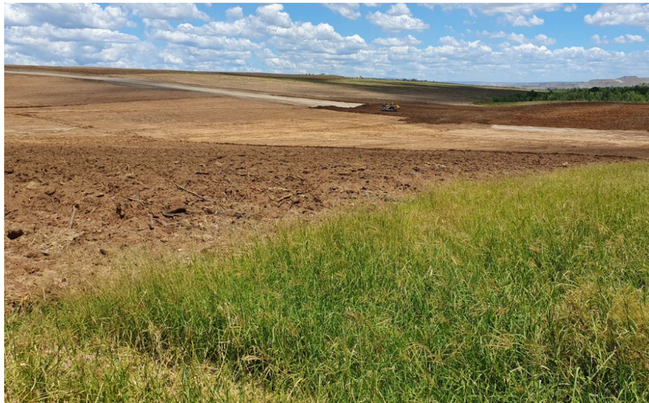
Figure 1 Example of topsoil application on dozed spoil with a plot established the previous year evident in the foreground
