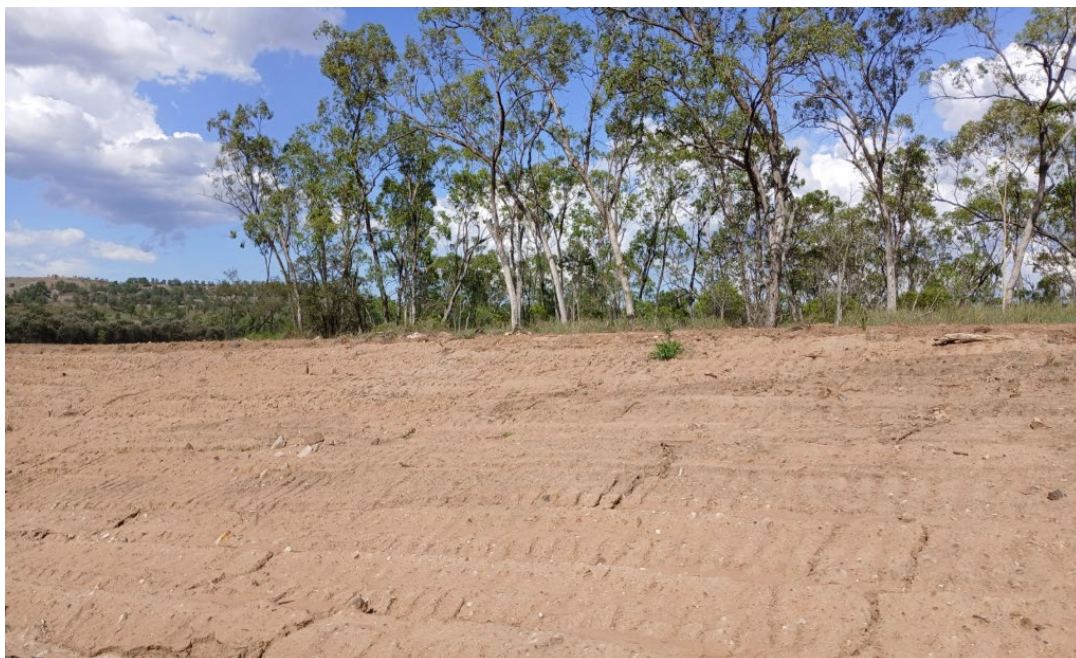
Figure 12 Cross ripped rehabilitation slope where the rip lines have failed to stop erosion and rills formed down the slope after a single rainfall event
