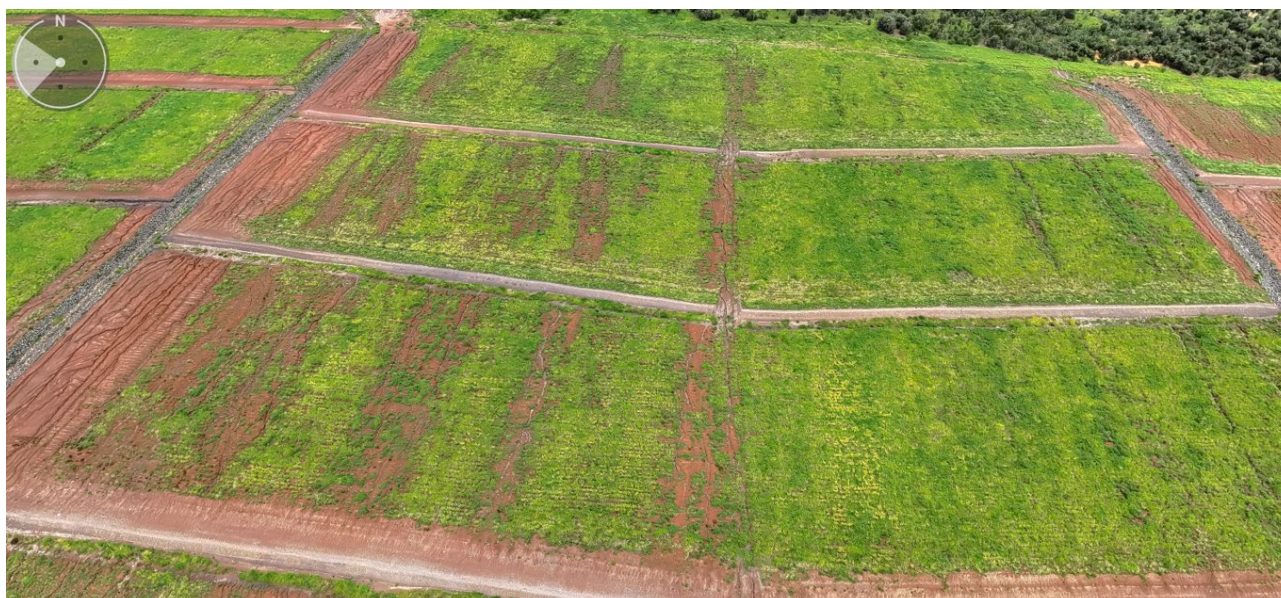
Figure 9 Recent topsoiled grazing PMLU with cross banks and spine drains after a single wet season
