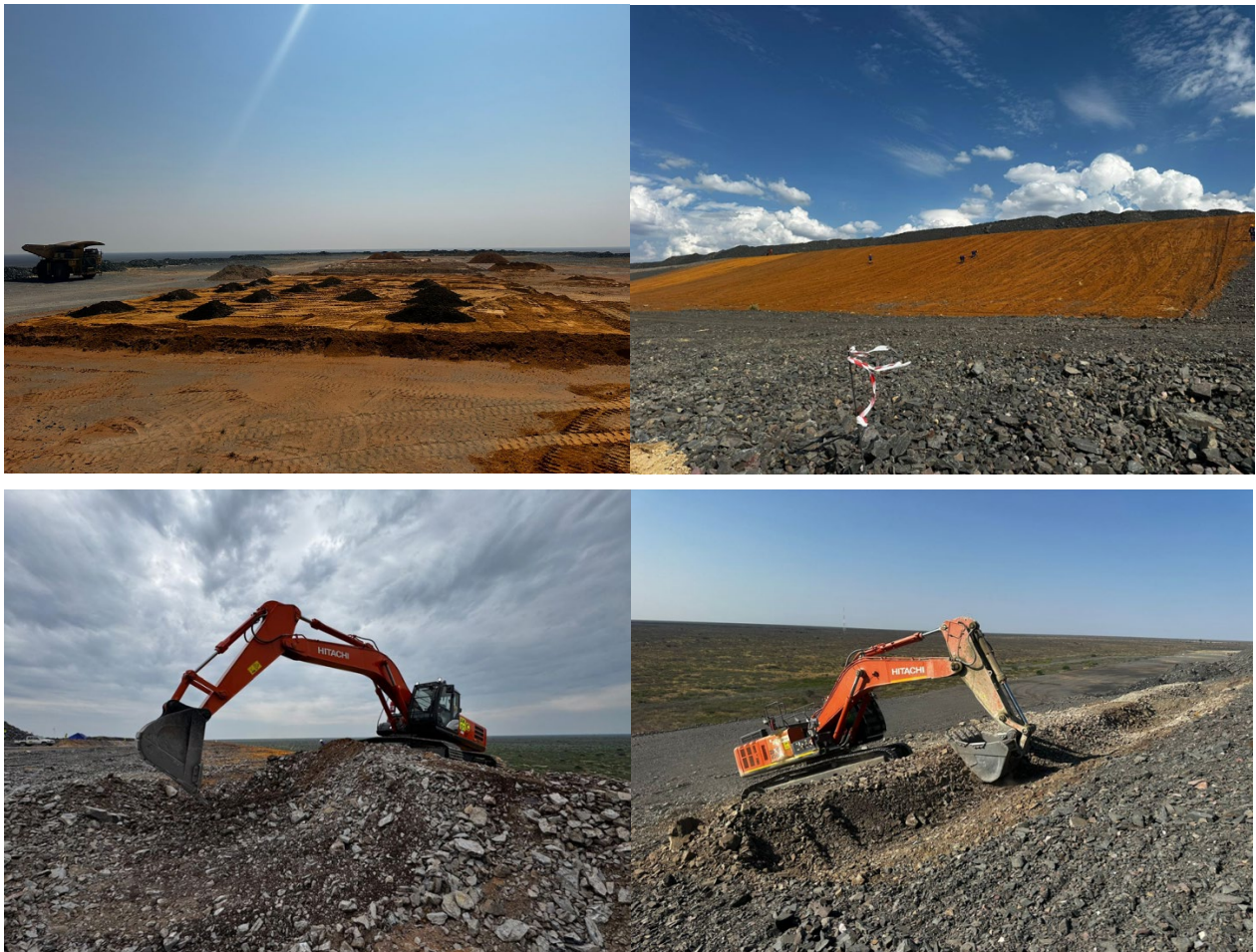
Figure 3 Implementation of trials (growth medium placement and stormwater structure construction)
