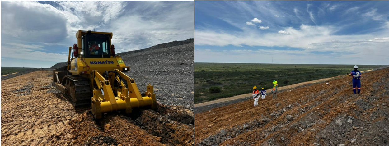
Figure 4 Implementation of trials (ripping and seeding)
