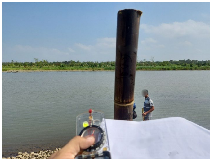
Figure 4 Boundary marker installation at a permitted sand mining site on the Progo River, with a compass survey in progress. Courtesy of PT Arsyandendra Panca Energi
