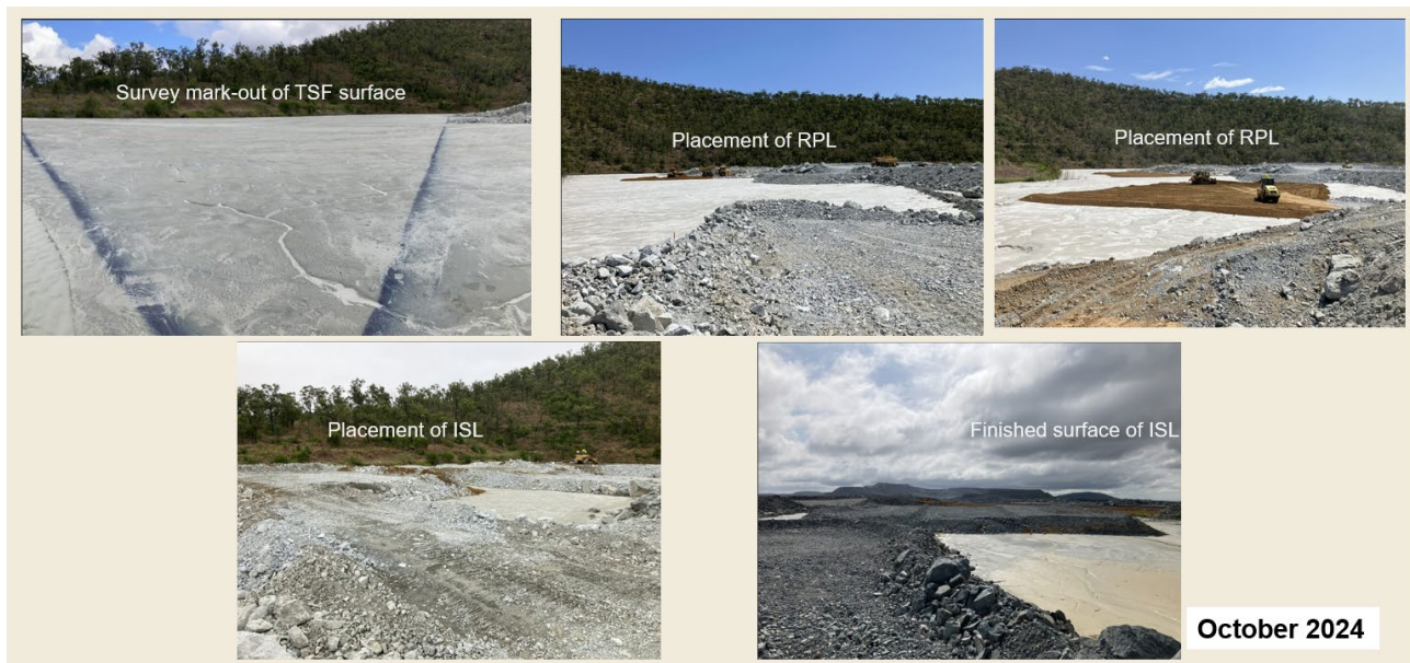
Figure 5 Sequence of trial pad construction
