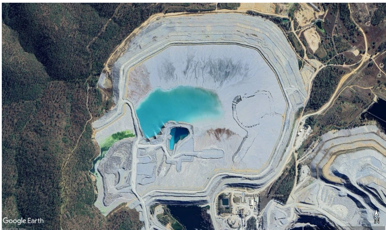
Figure 1 Aerial view of tailings storage facility at Mount Rawdon Operations
