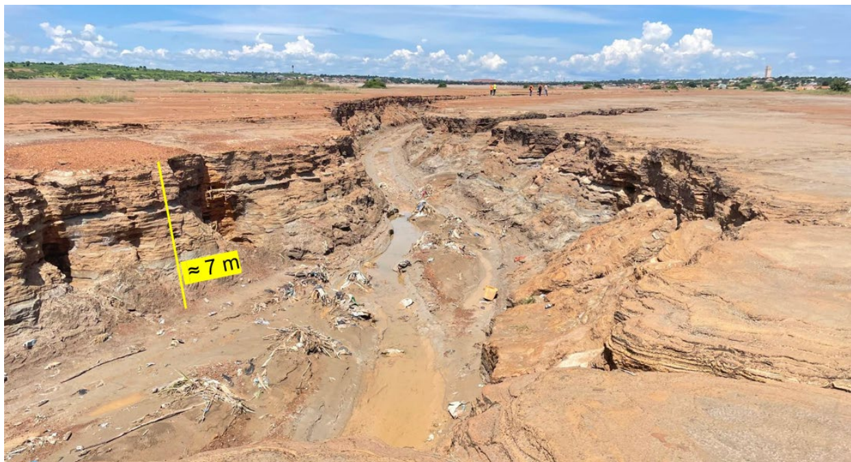
Figure 8 Eroding legacy tailings deposit near Kipushi in the Congolese Copperbelt
