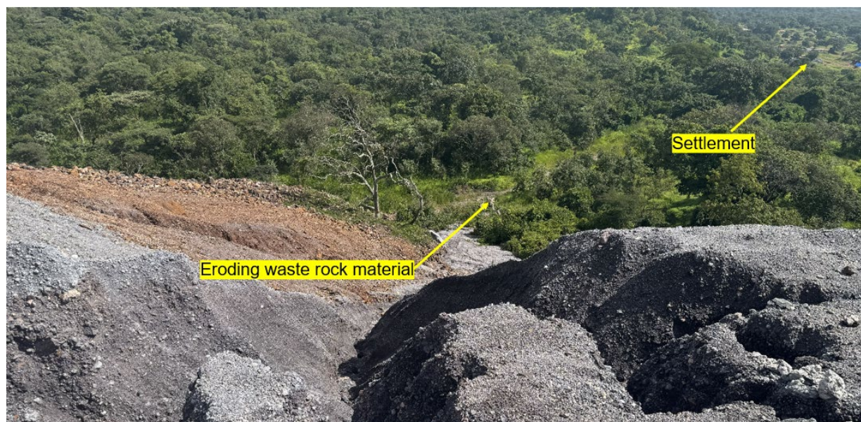
Figure 9 Eroding waste rock dump observed during field visits in the Congolese Copperbelt. Eroded material is mobilised downslope and deposited in a nearby stream channel flowing through the village
