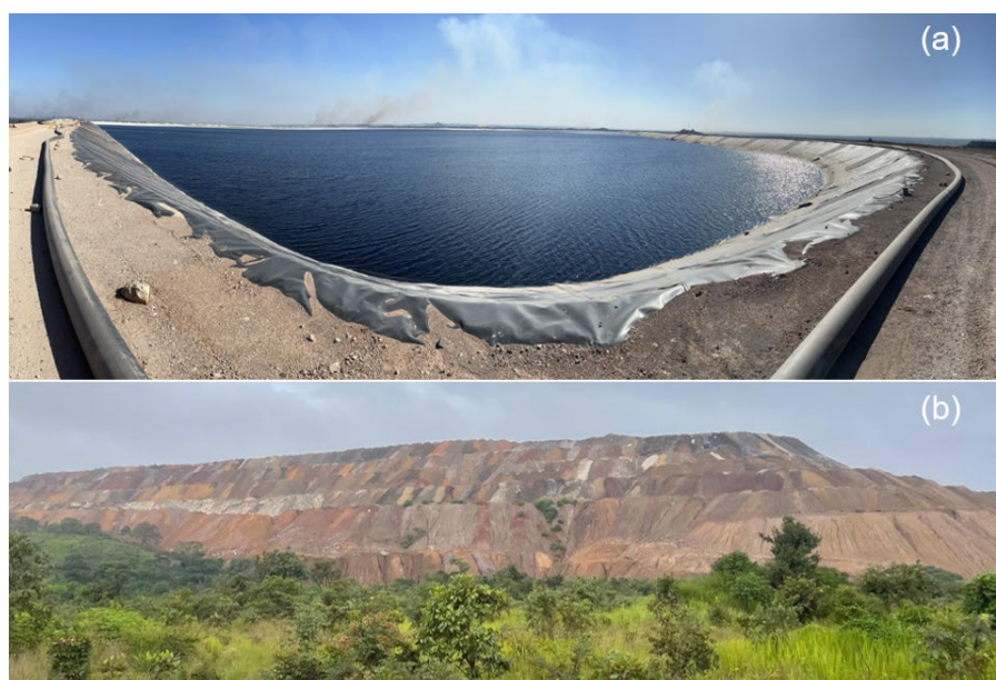
Figure 2 Examples of mine waste facilities observed during field visits in the Congolese Copperbelt. (a) A tailings storage facility; (b) A waste rock dump
