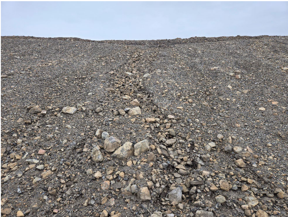
Figure 3 Self armouring on fill slope at an Arctic mine site
