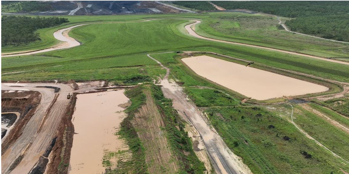
Figure 3 Recently constructed diversion exhibiting alluvial low-flow channel performance developing morphologic heterogeneity within a threshold high-flow channel in close proximity to an open cut pit
