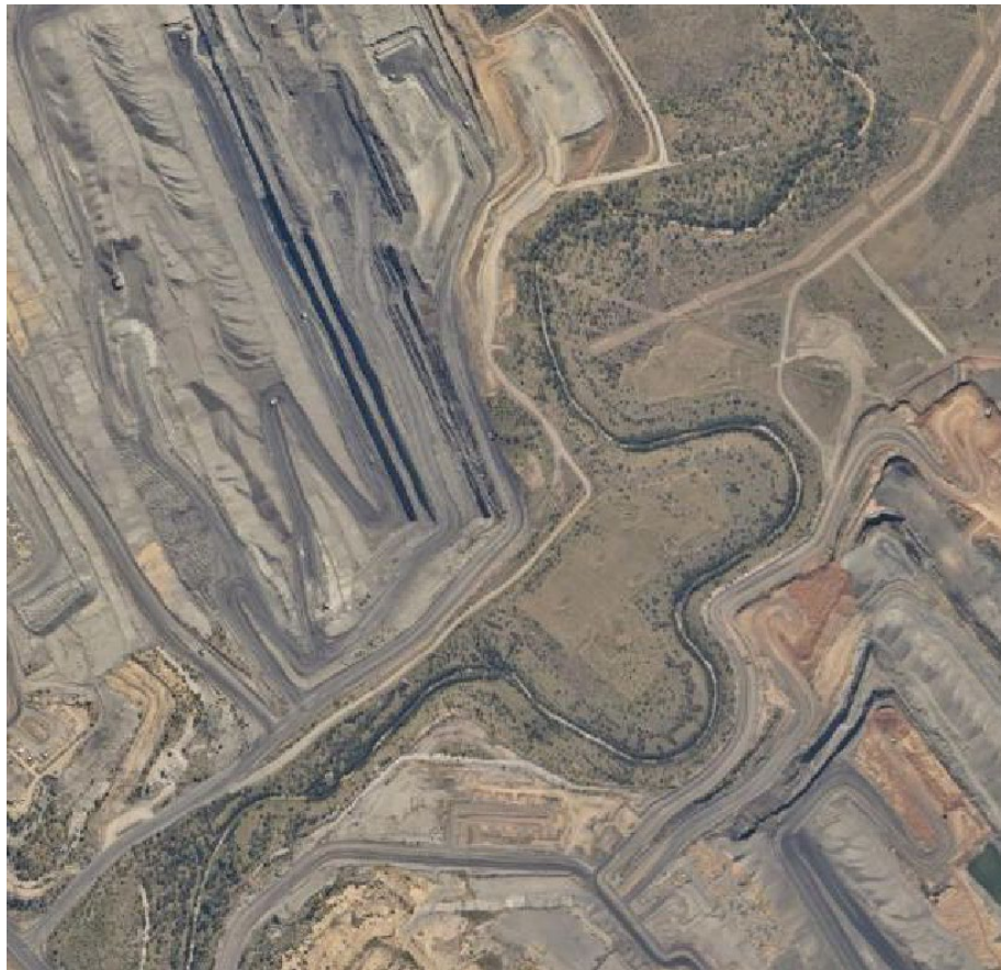
Figure 7 Aerial view of the ‘very good’ condition diversion in Figure 6, illustrating proximity to mining pits and dumps and the potential consequence of any channel migration
