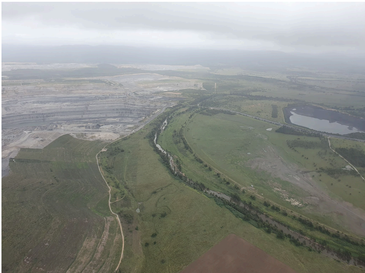
Figure 5 Low sinuosity alluvial channel directly adjacent to an open cut mine pit, illustrating the lack of potential for adjustment without severe consequences
