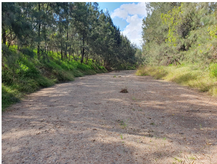
Figure 6 Diversion designed and constructed to the ACARP C20017 Standard, now 20 years old and in ‘very good’ condition
