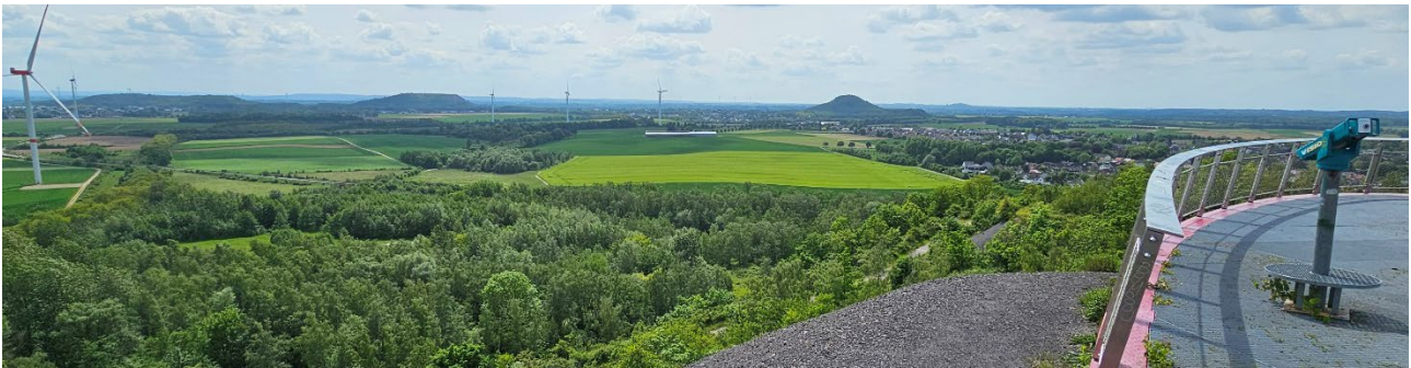
Figure 4 View from a coal spoil heap towards other revegetated coal waste dumps in the distance (Carl-Alexander waste dump, North Rhine-Westphalia). There are over 300 spoil heaps and landscape structures in North Rhine-Westphalia. Today, all sites have been closed and repurposed, and many of these landscapes now offer nature trails, magnificent views and landmark art on the summits of revegetated hills in the middle of the largest metropolitan region in Europe
