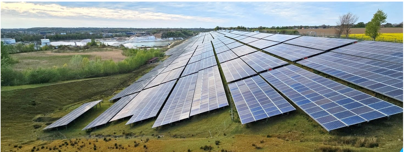
Figure 8 Solar park on a quartz sand-producing quarry (Nivelsteiner Sandwerke, North Rhine-Westphalia). The solar park currently produces renewable energy for around 5,000 homes nearby. The concept is to be expanded to include floating photovoltaic systems, wind turbines, batteries, combined heat and power plants, gas and steam power plants, and heat and hydrogen storage facilities to provide renewable energy to 50,000 people by 2030
