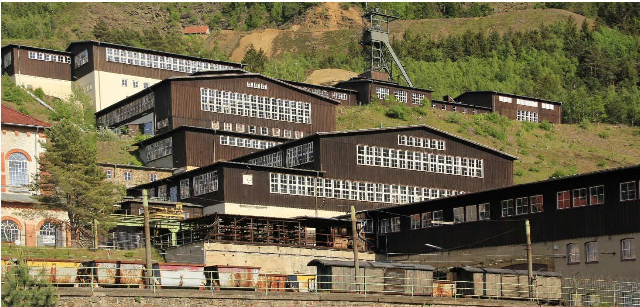
Figure 3 The historic Rammelsberg copper, lead, zinc, silver and gold mine operated for over 1,000 years (968 to 1988). It became a UNESCO World Heritage Site in 1992, and now attracts over 100,000 visitors per year
