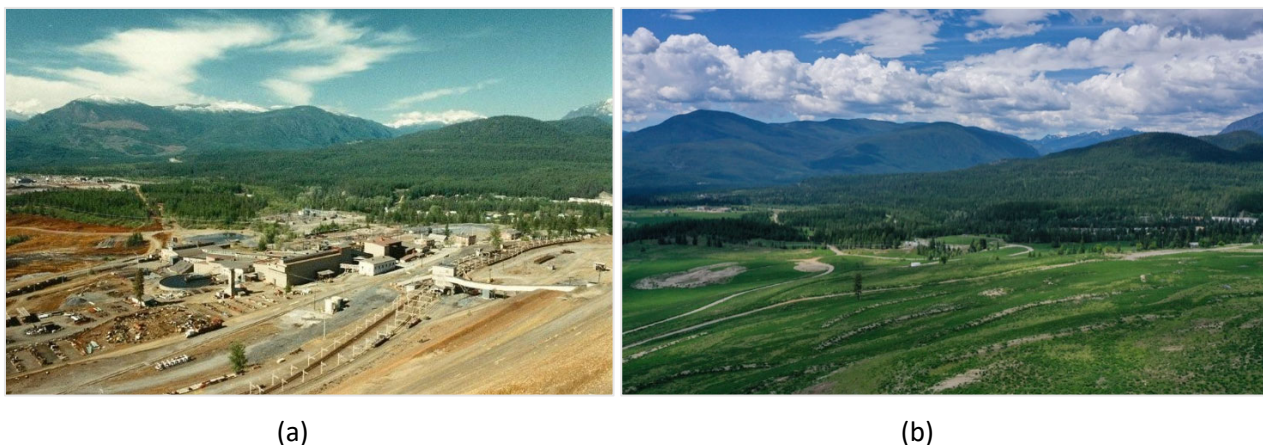
Figure 4 (a) Concentrator area at the Sullivan Mine during operations in 1989; (b) After implementation of post-mining strategies in 2020
