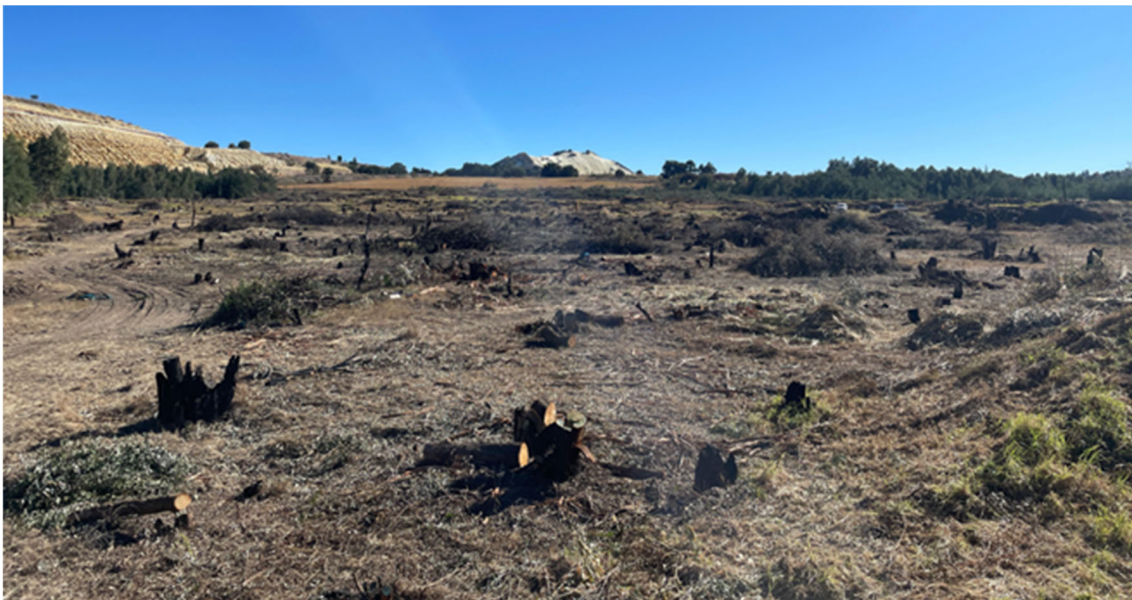
Figure 3 Site conditions in parts of the project area during the initial alien plant clearing by various contracting teams
