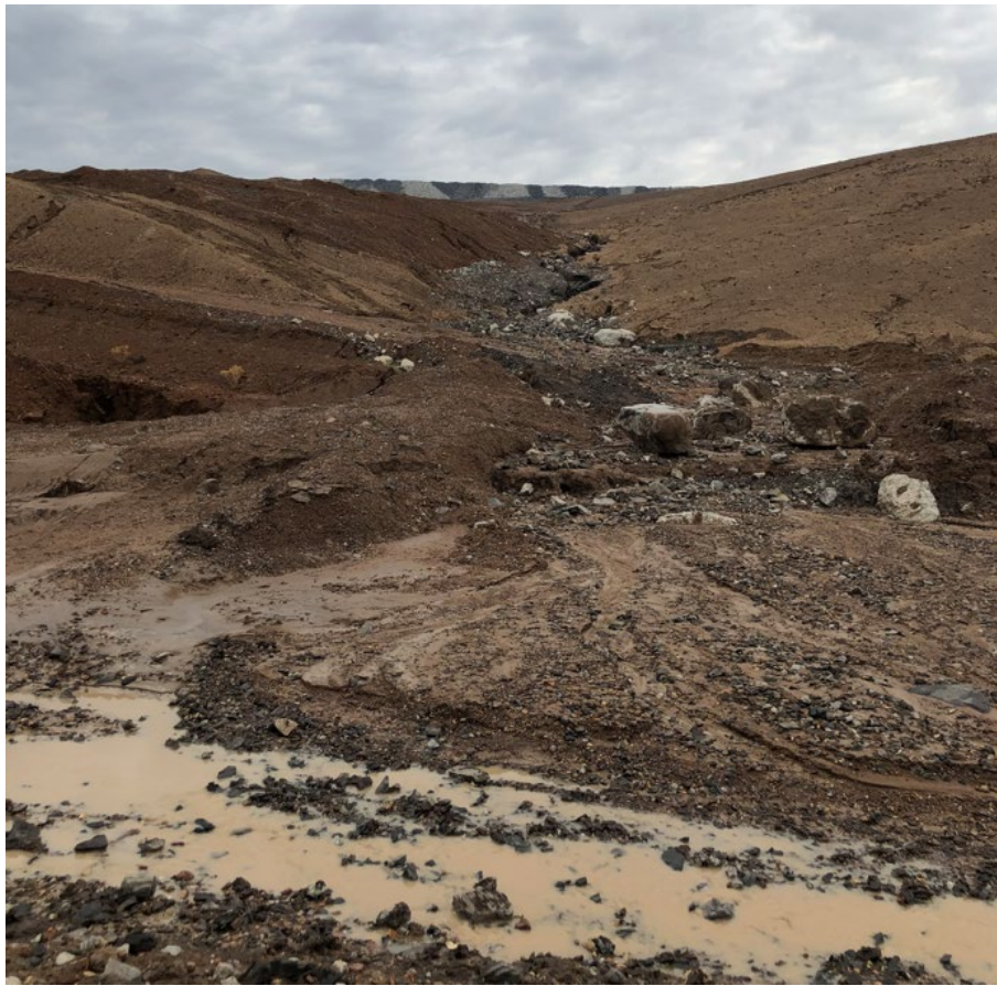
Figure 4 Status of the geomorphic landform adjacent to the failed drainage structure following an intense summer storm (January 2020)
