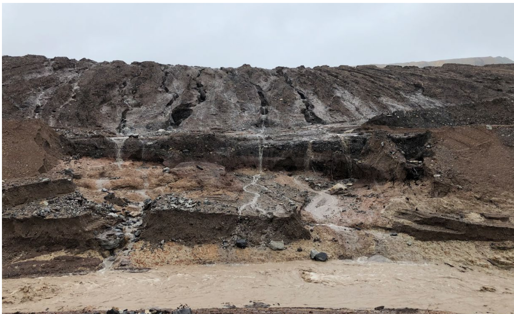
Figure 6 Erosion across the constructed geomorphic landform (following 8 February 2020 rainfall event)
