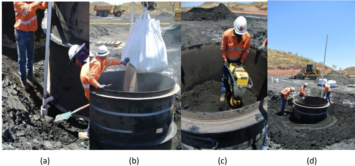
Figure 6 Lysimeter installation. (a) Sump; (b) Backfilling filter; (c) Internal compaction; (d) External compaction
