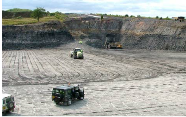
Figure 12 Daily impact rolling of 250,000 m 3 of coal spoil (Landpac)
