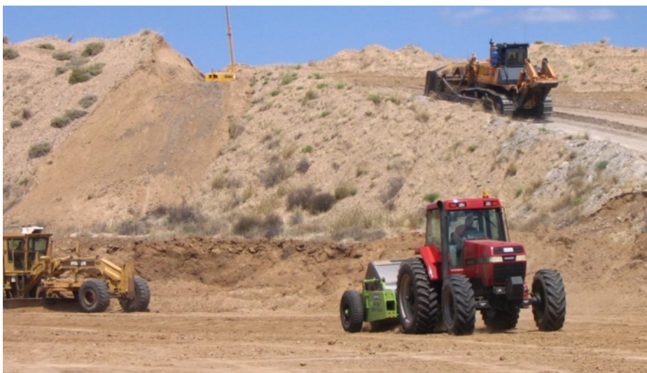
Figure 21 Impact rolling capping layer
