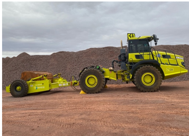
Figure 16 Impact rolling trial for tailings dam construction
