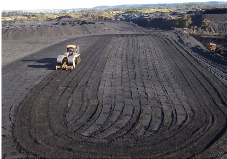
Figure 20 Impact rolling the coal washery reject to reduce voids and permeability
