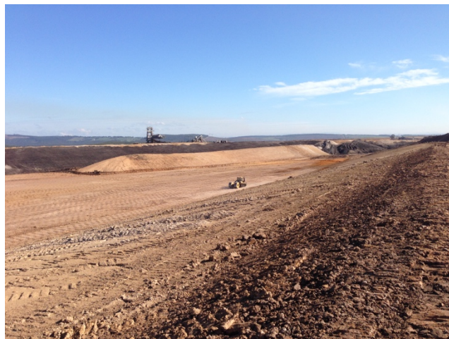
Figure 25 Ash containment cell impact rolling
