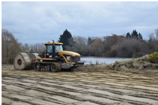
Figure 13 Impact rolling of coal overburden in 1.2 m layer thicknesses
