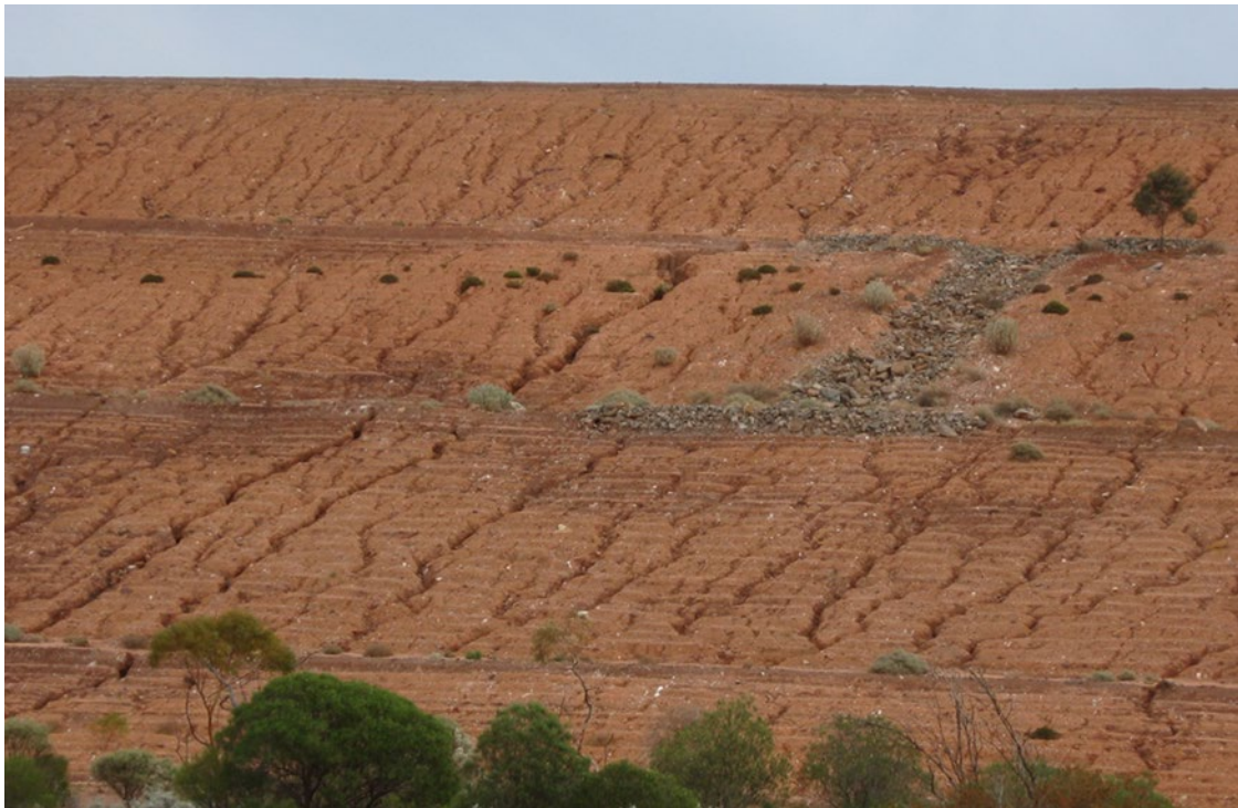
Figure 2 Rill development at consistent spacing across a landform batter on a waste dump in the WA Goldfields Region, 17 November 2004
