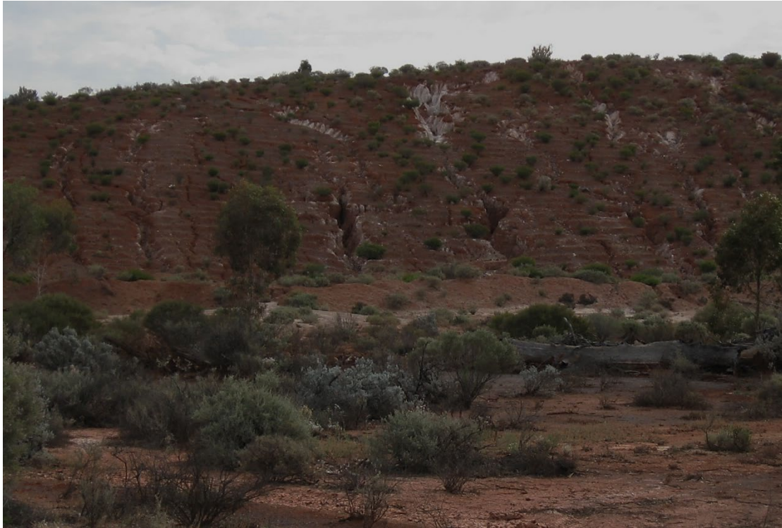
Figure 3 Gully development at consistent spacing across a landform batter on a waste dump in the WA Goldfields Region, circa 2005
