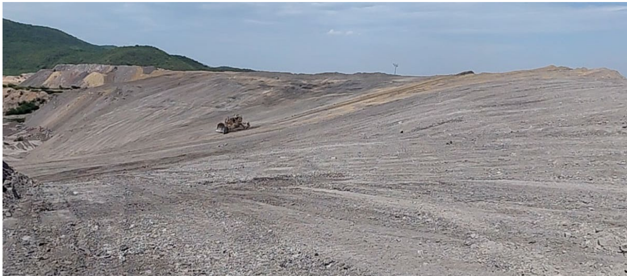
Figure 9 Tipiala ('Jaguar') geomorphic landform design scenario under construction (May of 2026) showing lifts being reshaped into 'natural' landforms. See Figure 8c for comparison and Figure 10 for the design
