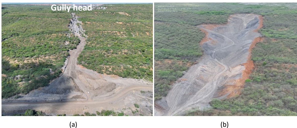
Figure 7 (a) Large gully at the Potrerito waste rock dump, formed by the overtopping of the dump's upper surface (gully head also shown in Figure 6a); (b) Initial geomorphic reshaping
