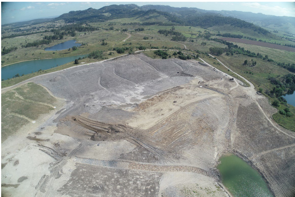
Figure 2 Antienne spoils capping viewed from the west during construction
