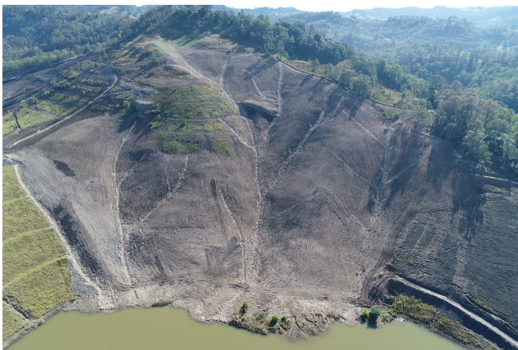
Figure 5 Mountain Block during construction viewed from the southwest
