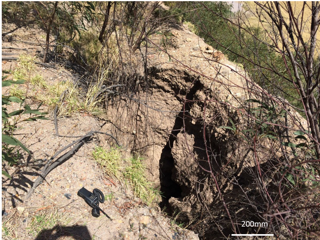
Figure 8 Piping failure at Liddell associated with the initial contour bank rehabilitation
