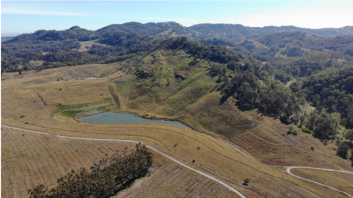
Figure 6 Mountain Block post geomorphic construction viewed from the south
