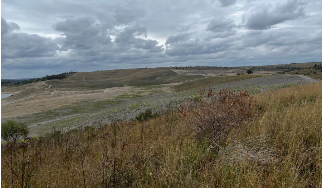
Figure 3 Antienne spoils capping viewed from east the during construction
