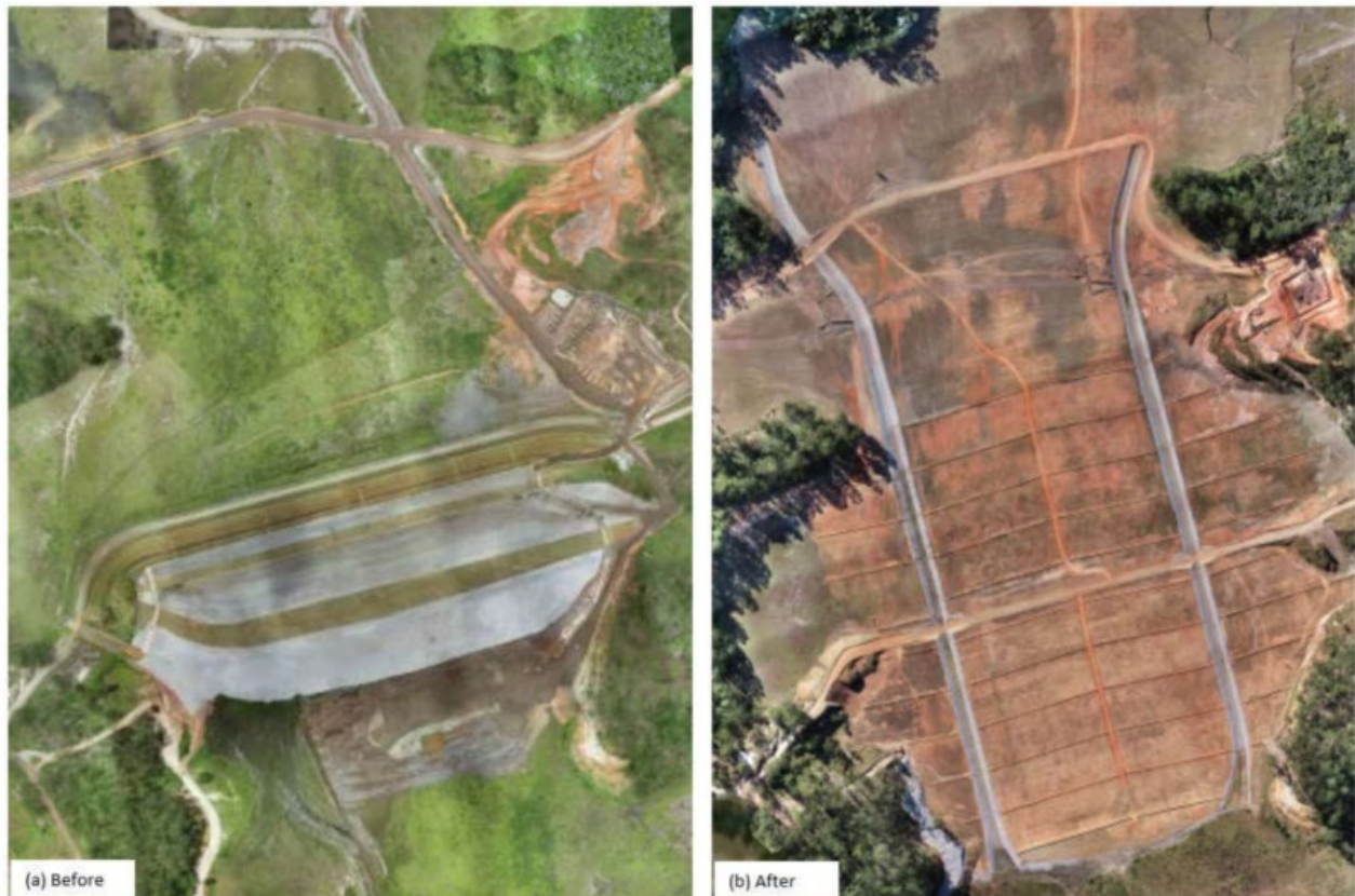
Figure 5 Orthophotos; (a) Before decommissioning works; (b) After decommissioning
