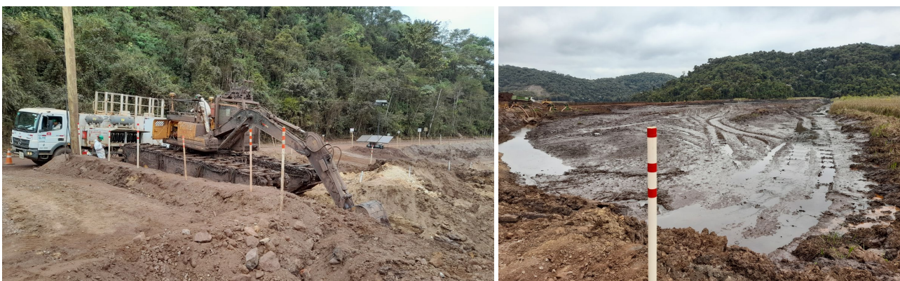
Figure 3 (a) Amphibious excavator; (b) Saturated tailings
