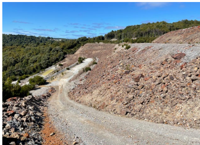
Figure 1 Mt Bischoff Happy Valley waste rock dump and an example of its steep slopes
