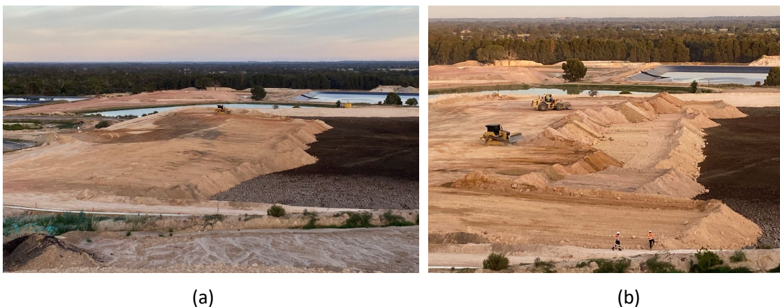
Figure 9 Photos showing placement of cover soil on Cell 1
