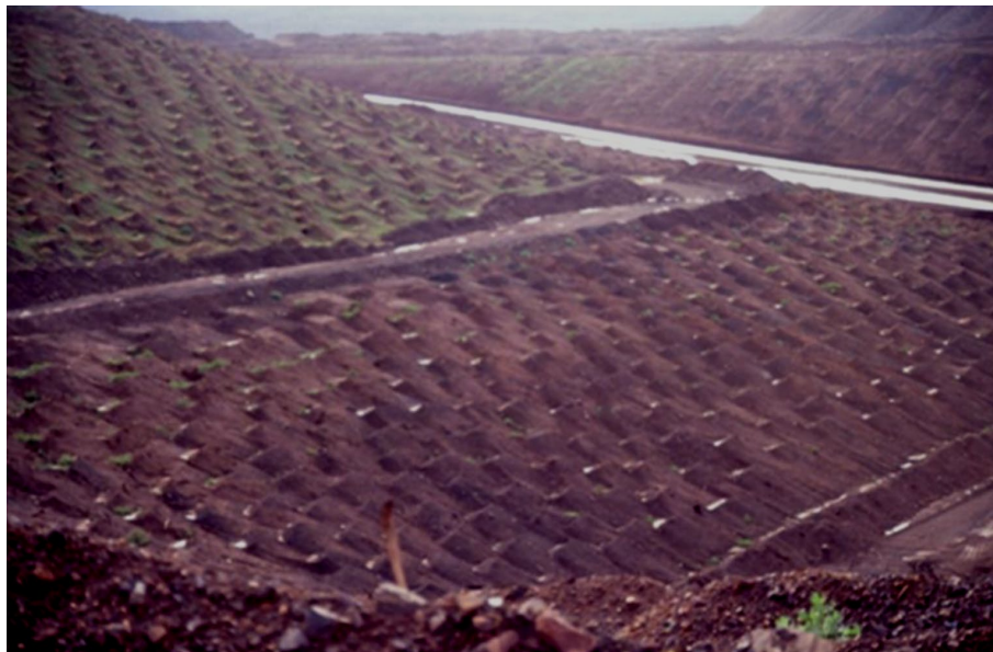
Figure 1 Successful moonscaping in Western Australia, iron ore mine, after a major cyclone (Note: Photo taken by H. Jones in 1978 as presented in Jones et al. [2012])
