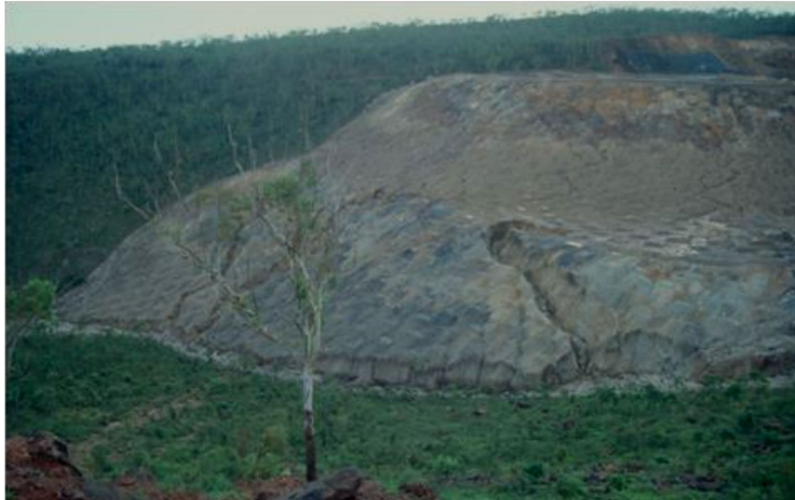
Figure 2 Failed moonscaping in northern Western Australia in the first wet season after construction, iron ore waste dump (Note: Photo taken by H. Jones in 1998 as presented in Jones et al. [2012])
