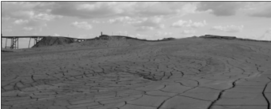
Figure 6: A 'finger dyke' supports the discharge pipe.
