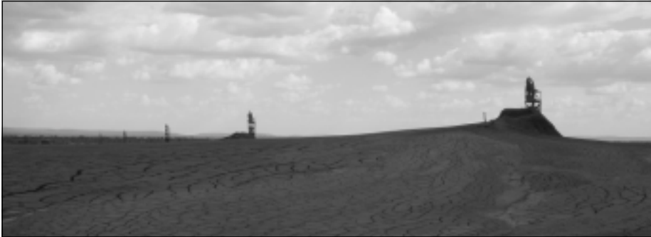
Figure 1: Five towers on TSF Cell 2, commissioned in August 2003.
