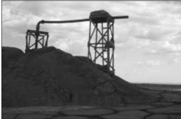
Figure 5: Horizontal tower extension, with wooden support tower.
