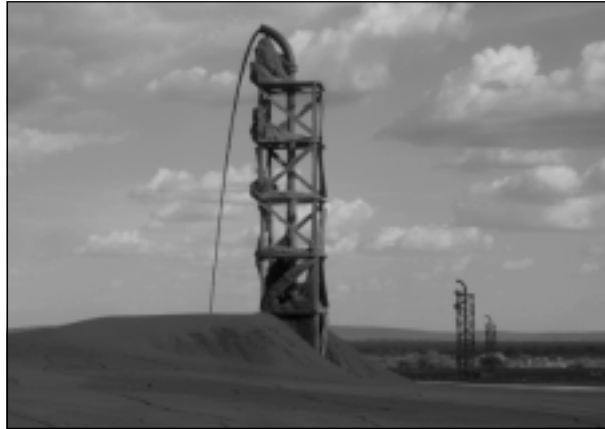
Figure 4: End of pipe discharge from a vertical pipe.
