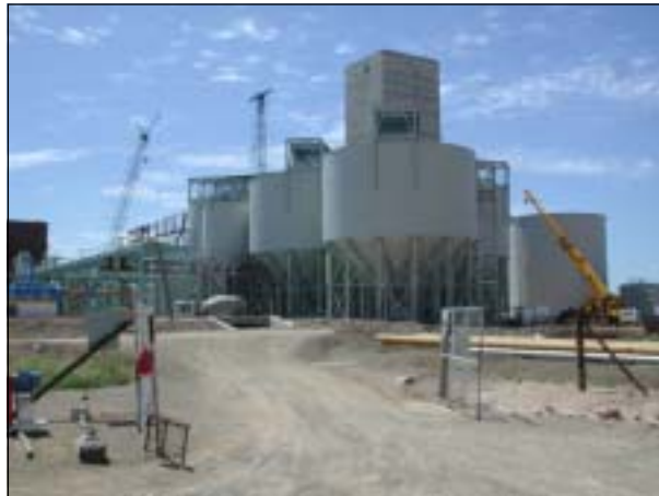
Figure 1: Multiple Deep Cone Thickeners.
