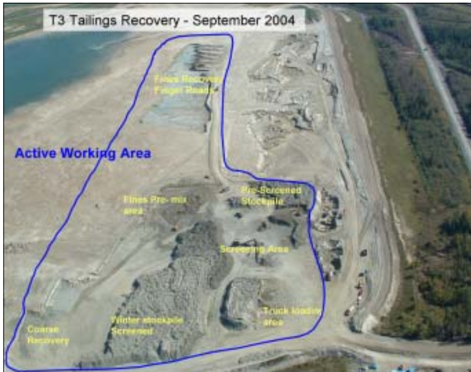
Figure 4: Overhead view of Tailings Area.
