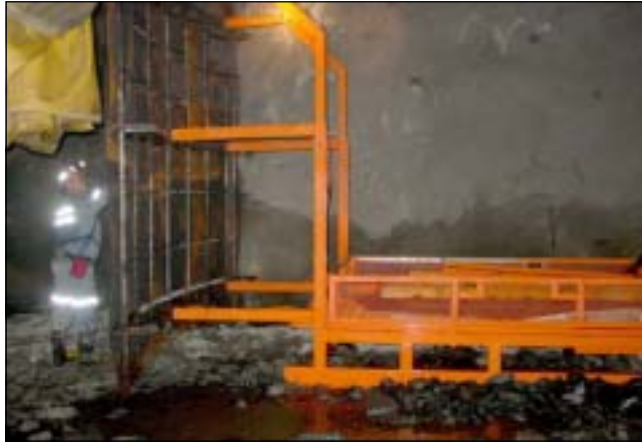
Figure 12: Shotcrete Bulkhead Construction.
