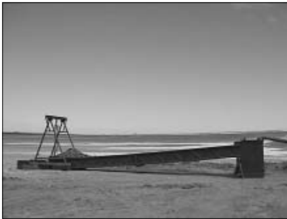
Figure 10: General view of the experimental flume installed at the mine site.
