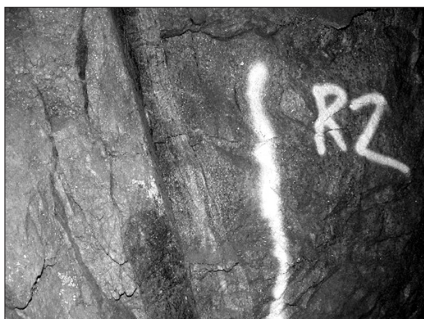
FIG. 2 R2-shear on 24 Level: Inspection revealed no sign of any slip having occurred on this structure
